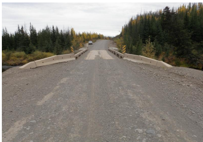
Figure 1-3: Looking towards camp end.
