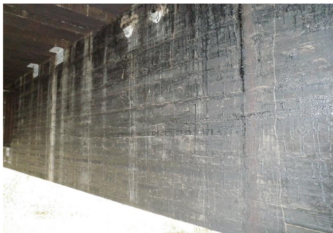
Figure 1-18: Girder 3 upstream face.
