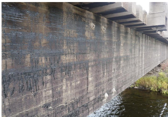
Figure 1-16: Girder 1 upstream face.
