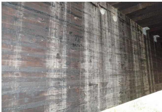
Figure 1-17: Girder 2 downstream face.
